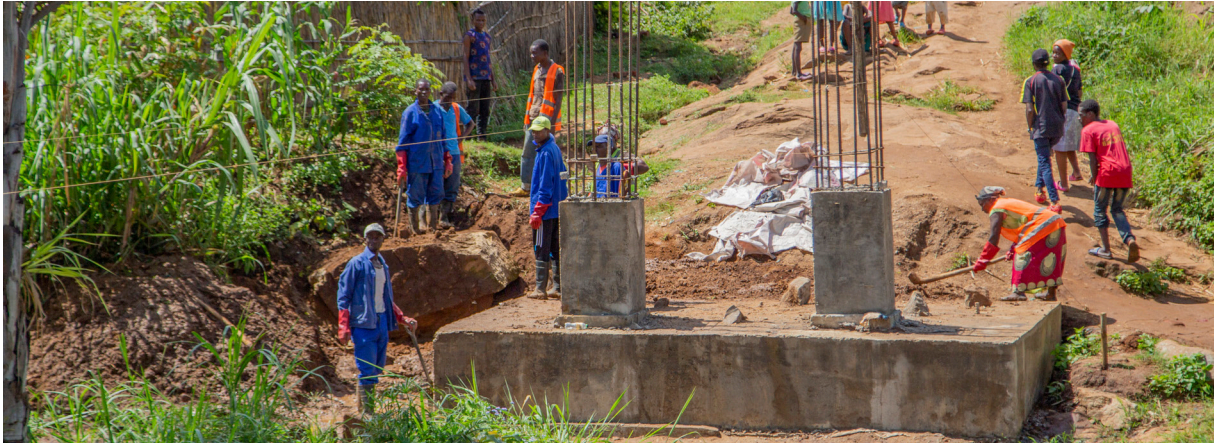
FIGURE 8 | The Linkgala Bridge construction site
