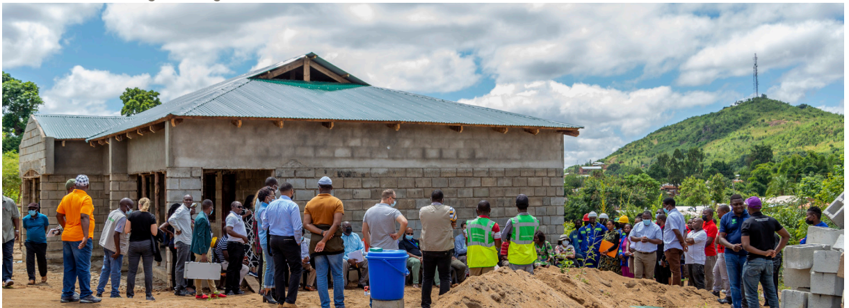
FIGURE 9 | Community members and project teams inspect the Linkgala evacuation center
