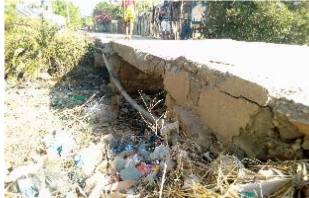
Current Photo of Bemokijy Bridge
