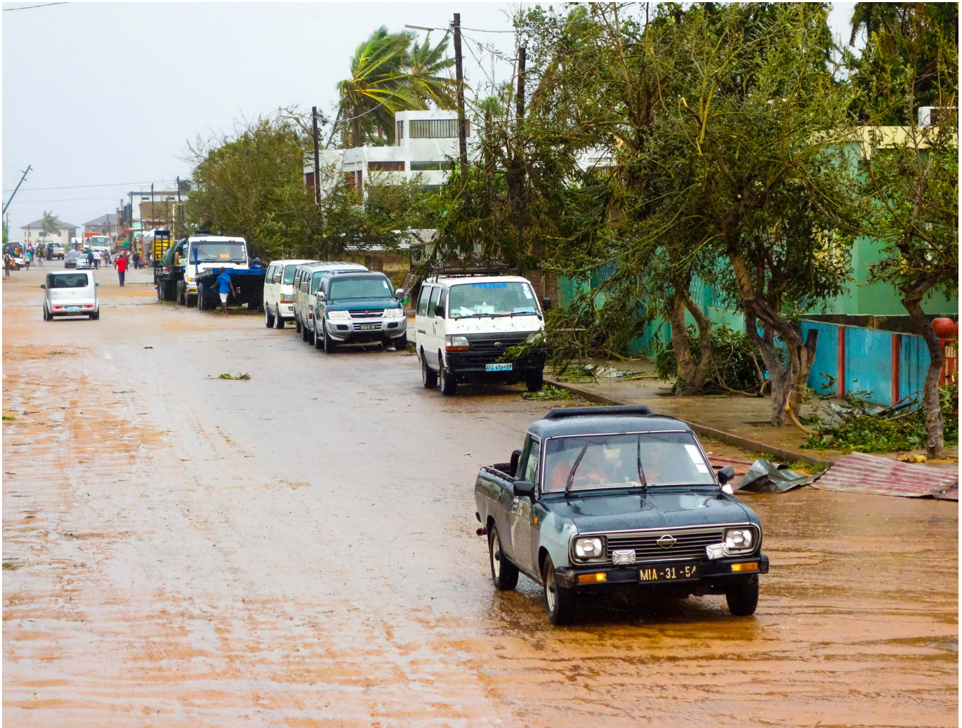
A tropical cyclone destruction at the center of Maxixe city, Mozambique © Shutterstock/Tonis Valing
