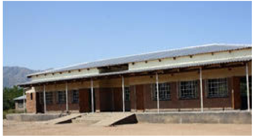
Figure 13: Elevated school and safe haven in Chikwawa, Malawi. UN-Habitat, Habitat for Humanity, DoDMA, funded by DIPECHO
