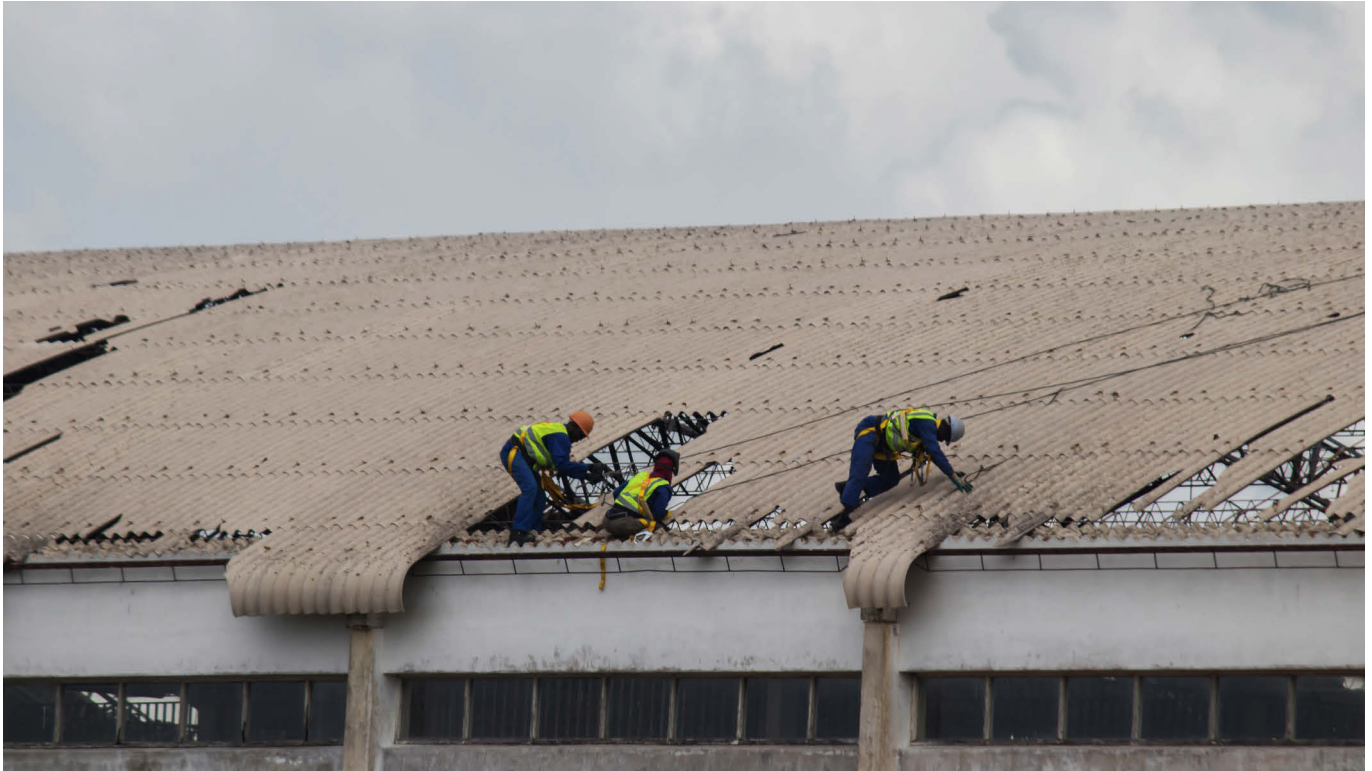
People fixing a damaged roof after a cyclone, Beira city, Mozambique © Shutterstock/MiroS Lav
