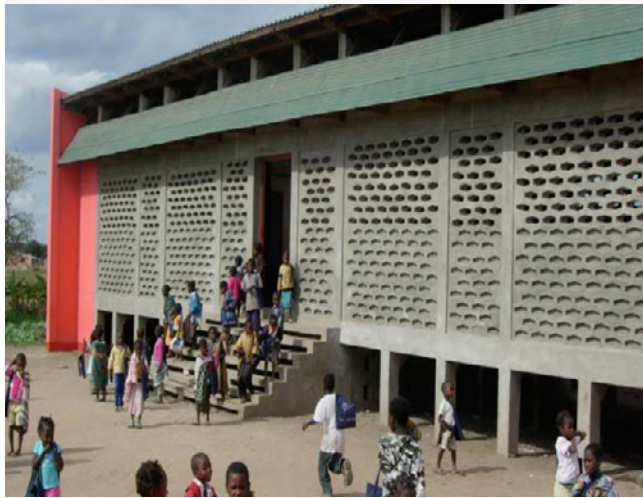
FIGURE 21 A, B Infrastructure of education. Elevated school construction protects from flooding. Reinforced school roofs protect from cyclones.
