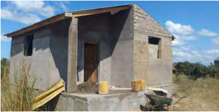
Photo: UN-Habitat - Construction process
