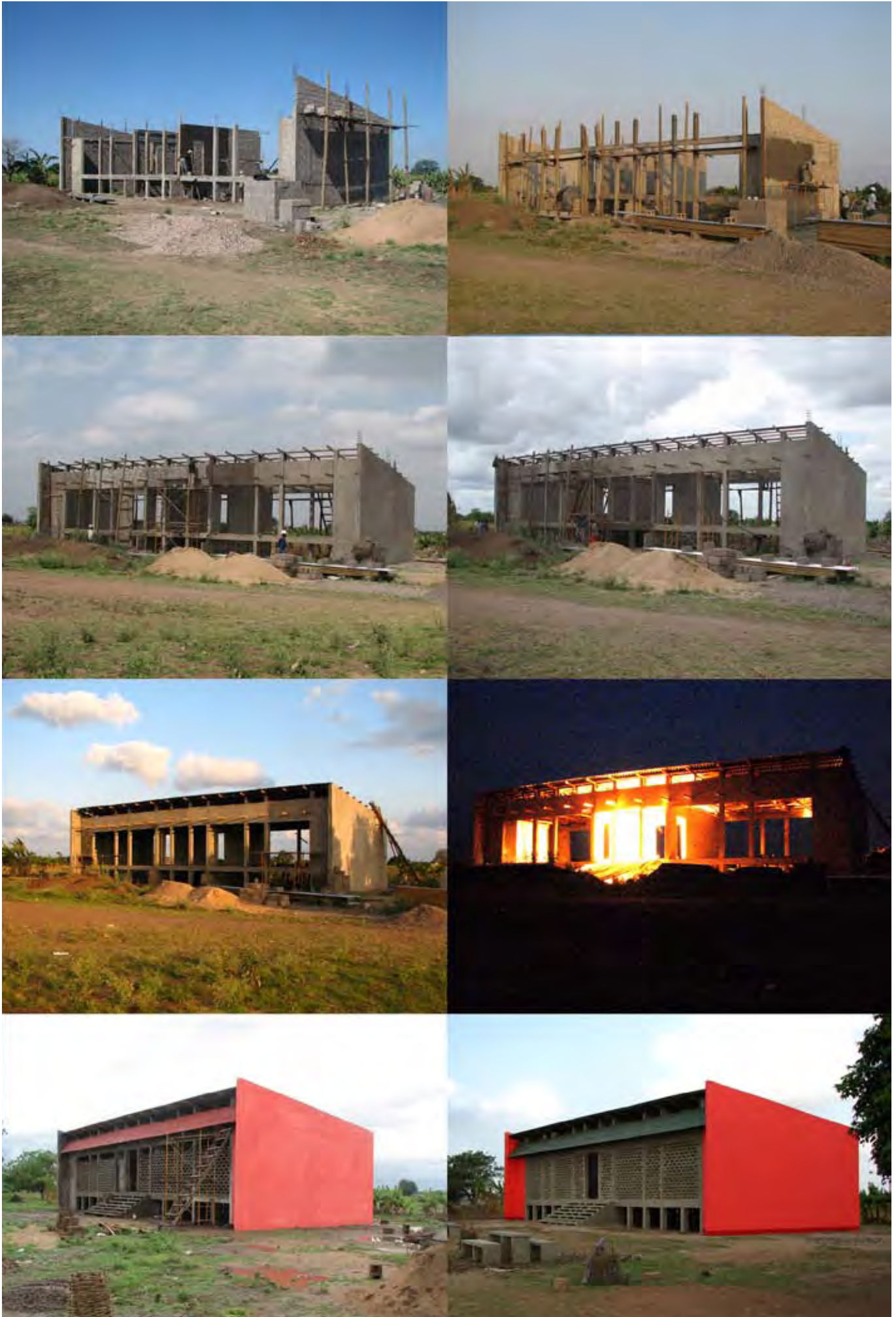
Photo: UN-Habitat - Construction Process
