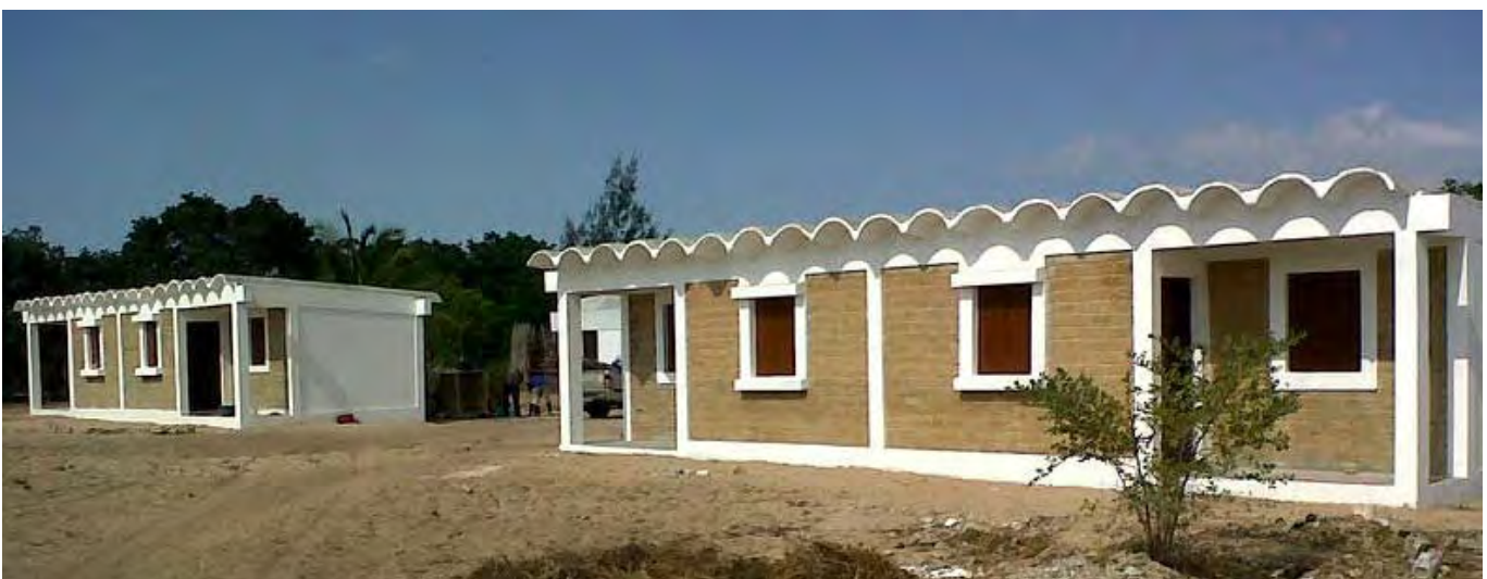
Photo: UN-Habitat - Houses covered with pre-industrialized ferro-cement vaulted roofing panels
