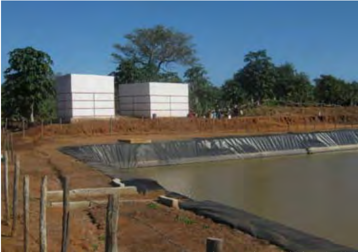
Photo: IRD - Water reservoir and concrete made units / Mabiñale, Massinga District
