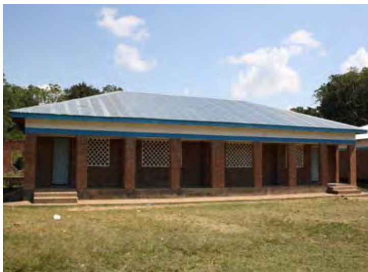
Photo: UN-Habitat - Surveyed Reconstructed School: Mwenitete Local / Karonga / S 09°48'46.1" - E 033°52'23.9'
