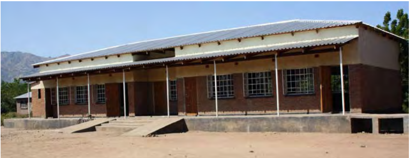
Photo: UN-Habitat - Safe Heaven: Nankapa Village / T.A. Makhwira / Chikwawa / S 16°17'41.3" / E 035°01'54.8"
