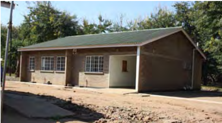
Photo: UN-Habitat, Makhira Health Centre, Chikwawa District / Staff House built with Stabilized Soil Blocks
