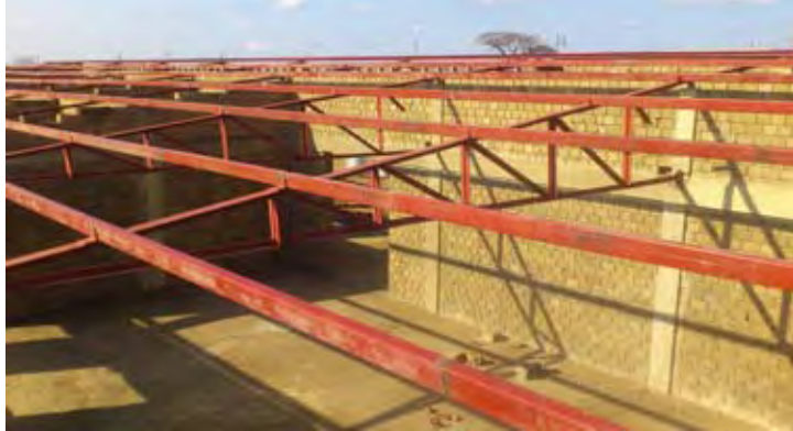
UN-Habitat - Main Building, construction process
