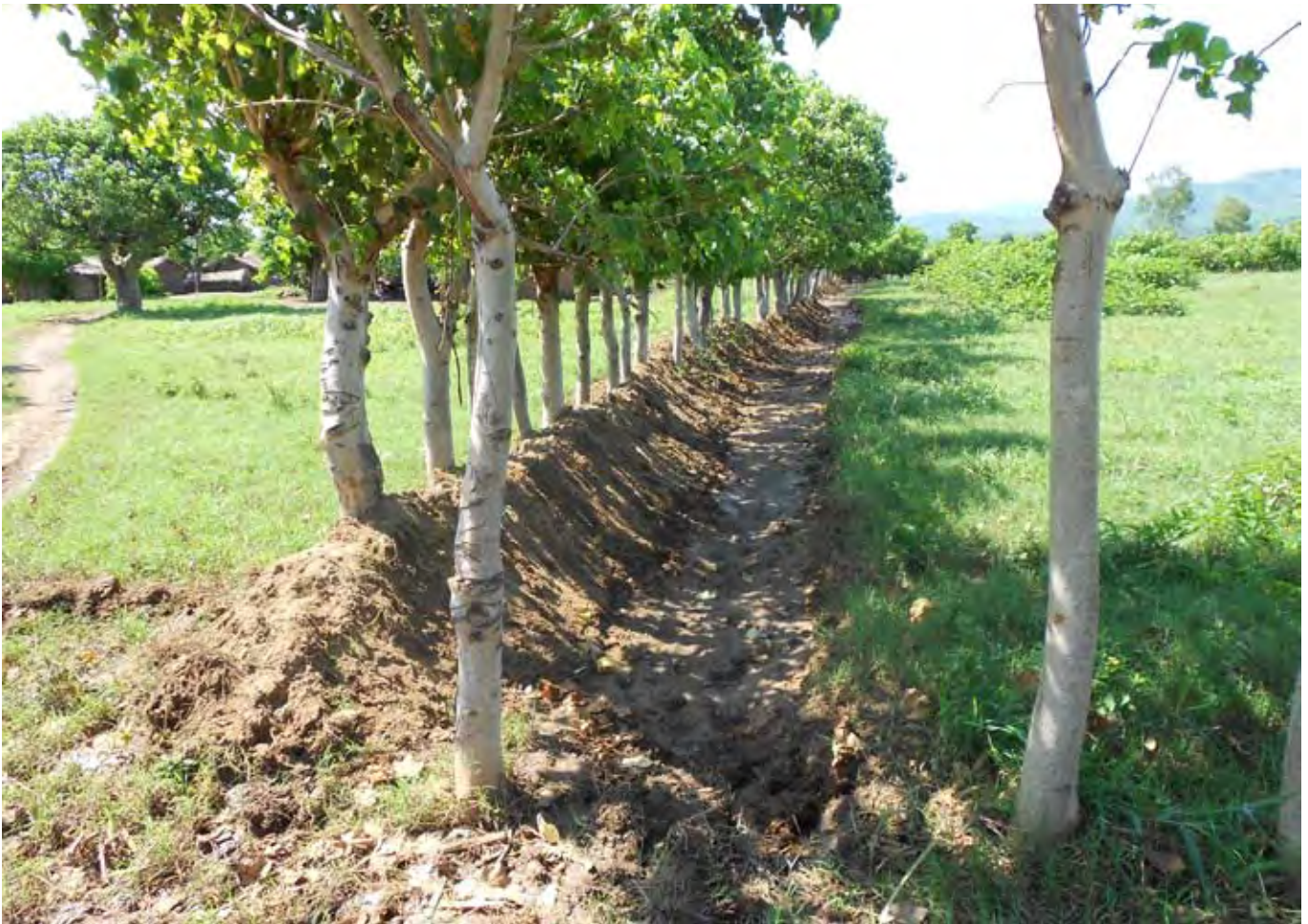
Photo: UN-Habitat, Community constructed drain, Jana Village
