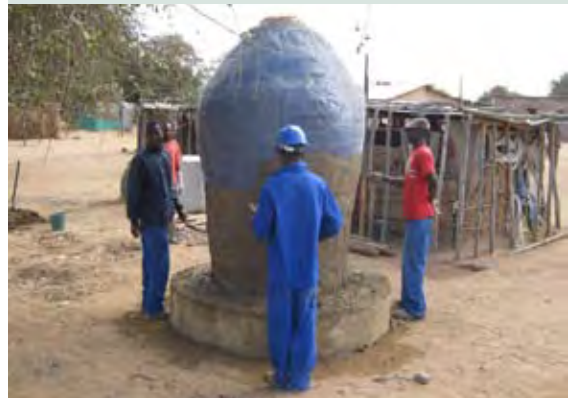
UN-Habitat - Ferro-Cement Tank Model 2, construction process
