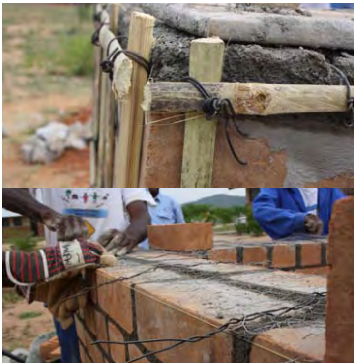
Photo: UN-Habitat - Wall Reinforcement Techniques: bamboo slats and metal wire
