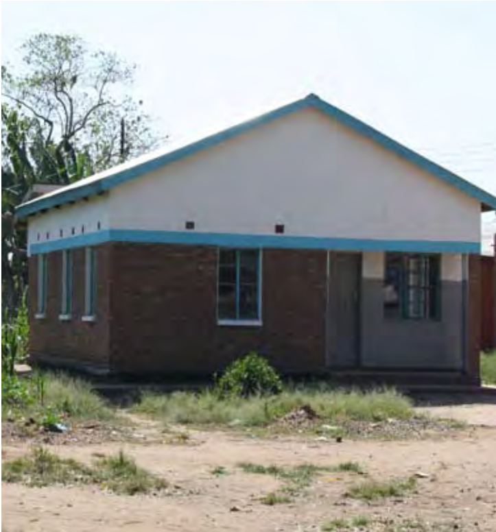
Photo: UN-Habitat - Surveyed Reconstructed School: Mwenitete Local / Karonga / S 09°48'46.1" - E 033°52'23.9'
