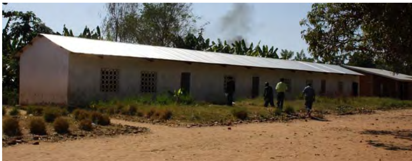
Photo: UN-Habitat - Surveyed Reconstructed School: Mwenitete Local / Karonga / S 09°48'46.1" - E 033°52'23.9'
