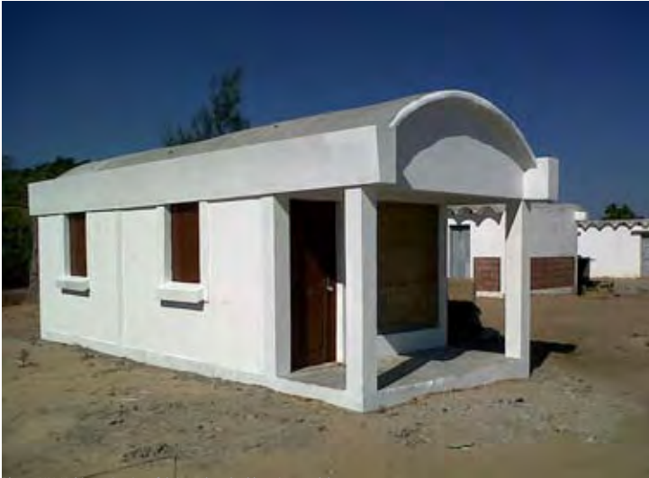
Photo: UN-Habitat - Semi-prelabricated vaulted housing model
