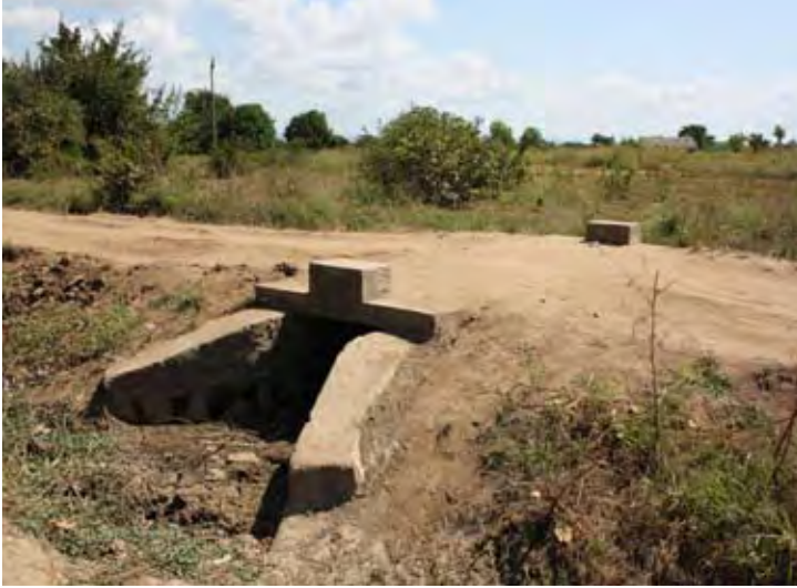
Photo: UN-Habitat - Surveyed Bridge: Mwenitete Local / Karonga / S 09°52'28.9" - E 033°53'46.1"
