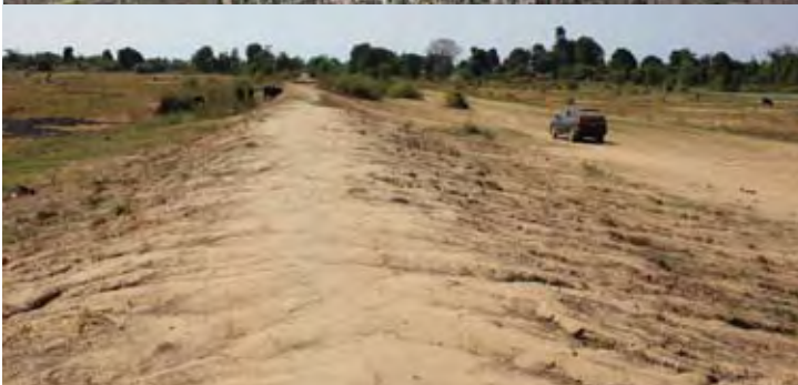
Photo: UN-Habitat - Rehabilitated Dike / Karonga / S 09°55'46.0" - E 033°55'15.1"
