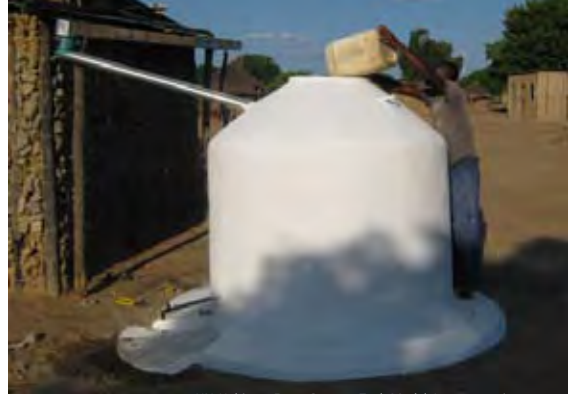
UN-Habitat - Ferro-Cement Tank Model 1, construction process
