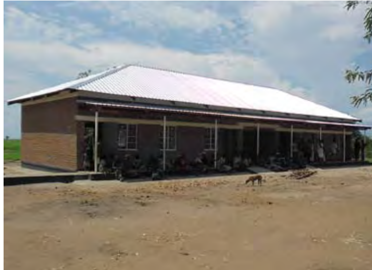
Photo: UN-Habitat - Surveyed Evacuation Centre: T.A. Ngowe / Chikwawa / S 16°30'50.2" - E 035°00'53.2"
